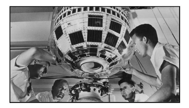
This image shows the mounting of the Telstar 1 satellite on the rocket that launched it into orbit. The satellite was ball-shaped and had its solar panels mounted around its exterior. Mounting the solar panels all the way around the satellite like this ensured that some solar panels would always be facing the sun.
